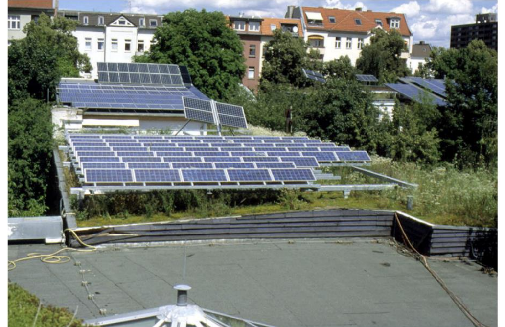
Figure 4: General overview of the different types of roofs (July 2001)
